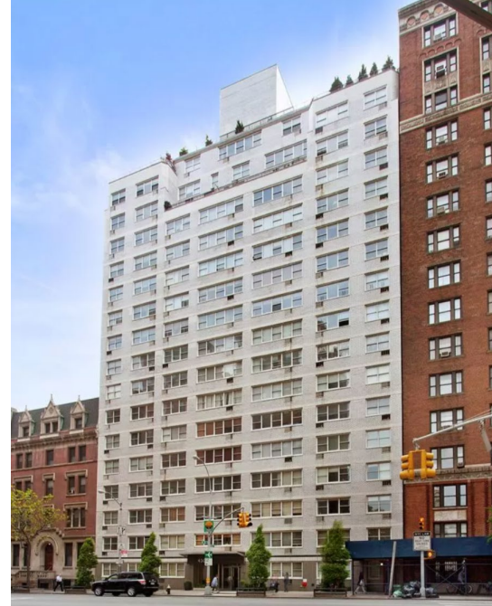
430 West 34 th St. MOD – Destination Dispatch (11) Gearless Traction Archstone Builders
