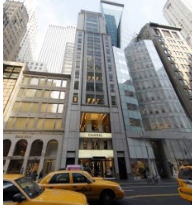
Chanel 15 East 57 th 3 Geared + 1 Gearless Traction Elevators Shawmut Design & Construction
