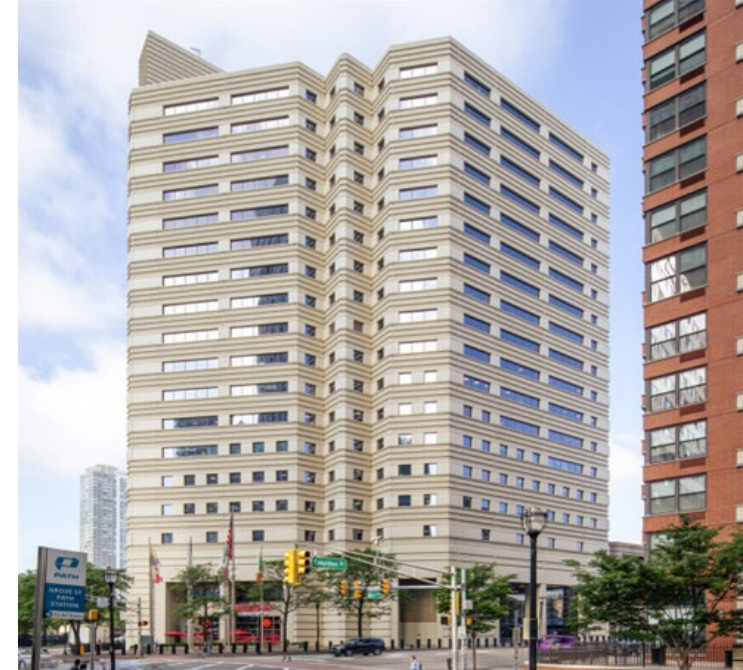
95 Christopher Columbus MOD – Destination Dispatch (11) Overhead Gearless Traction Wells REIT / Columbia Property Trust LLC
